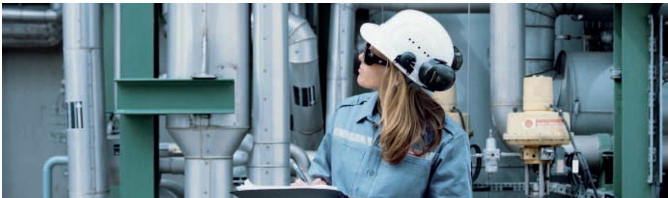
↳ CO 2 treatment unit for an environmental project at the Kwinana site, Western Australia
